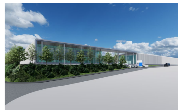
Miharu plant new building
