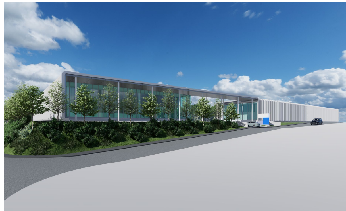
Expected exterior of Miharu new plant
